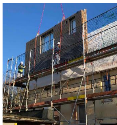
Prefabricated facades being used in a retrofit in Hameln, Germany. © Ecoworks
